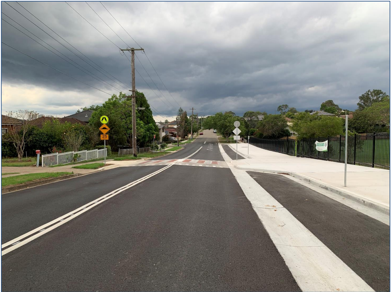
Figure 3.7: Northern zebra crossing on Smalls Road
